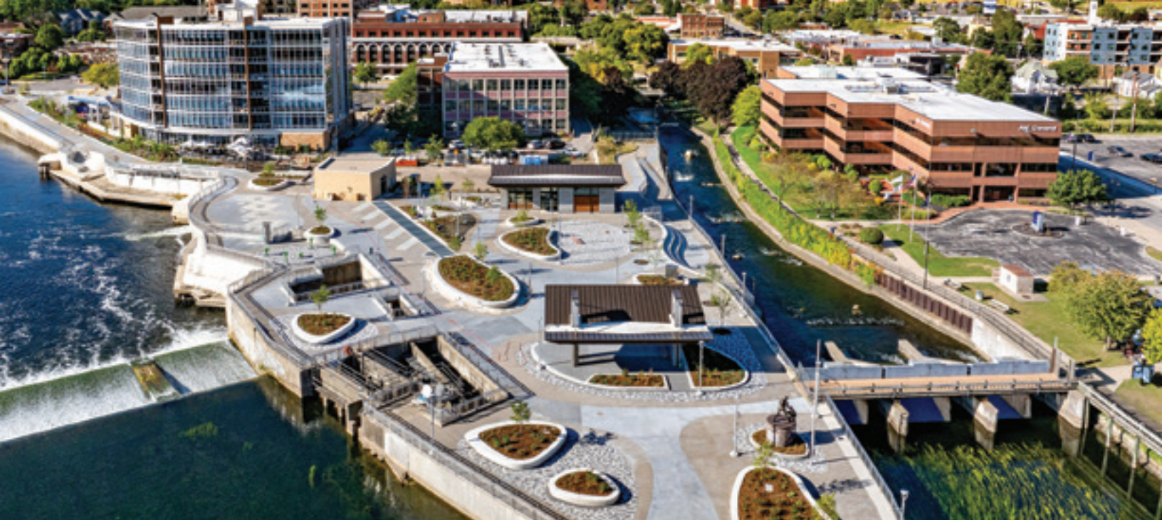
^ Pictured is Seitz Park along the St. Joseph River in South Bend. Underneath the park is a hydroelectric facility that generates power for campus. (Photo by Matt Cashore, University of Notre Dame)
